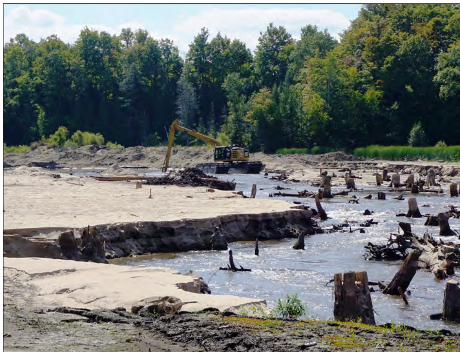
An amphibious trac-hoe works on excavating the relic channel through the former Sabin Pond. Photo courtesy of CRA
