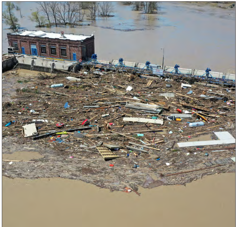
Debris build up near Sanford Dam after a 100-year flood caused a dam failure and severely damaged one other dam.
